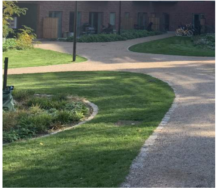
Water infiltreren in halfverharde hoven
